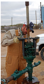
Install stuffing box protector
