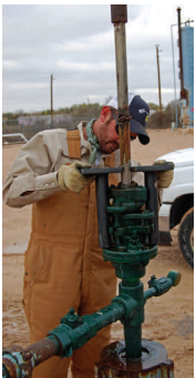
Install stuffing box protector
