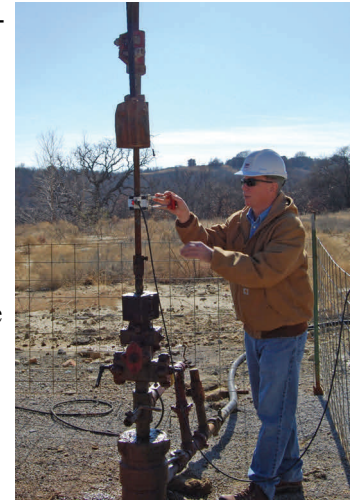
Installing Quick Clamp on rod string
